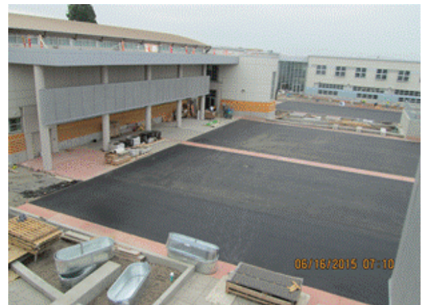
Site: Paving at courtyard areas.
