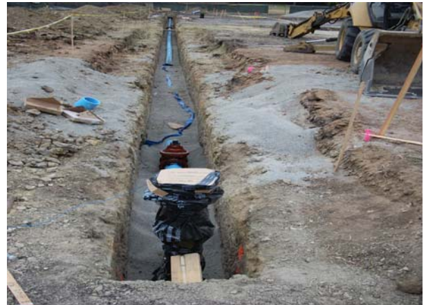
Underground fire water piping
