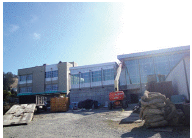
Building C - Exterior Painting
