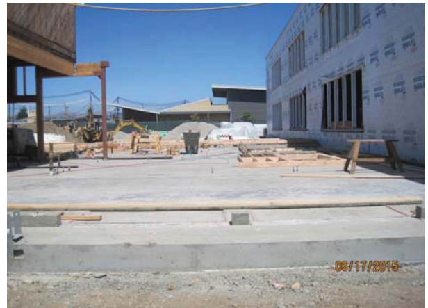
Administration Building Slab on Grade
