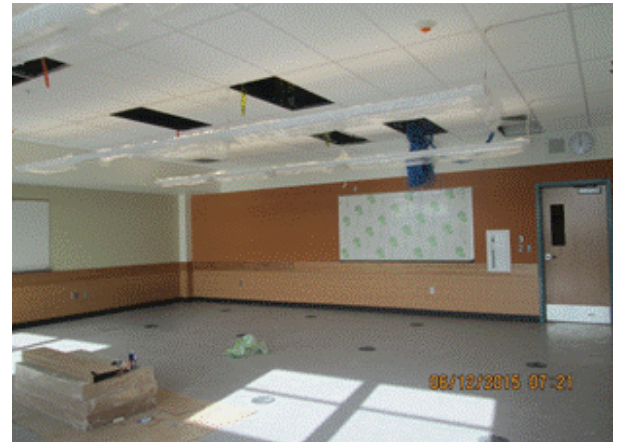
Building A - LPS: Stretched fabric at classroom walls.
