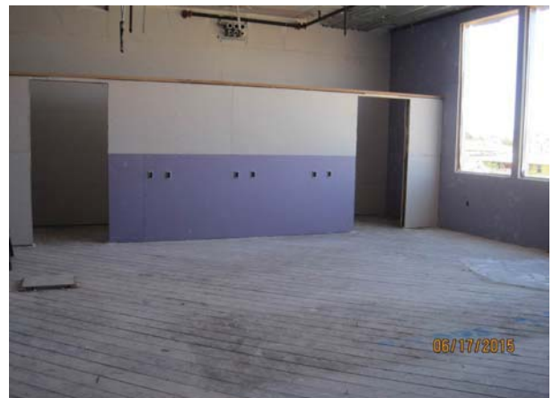
Typical Classroom Drywall
