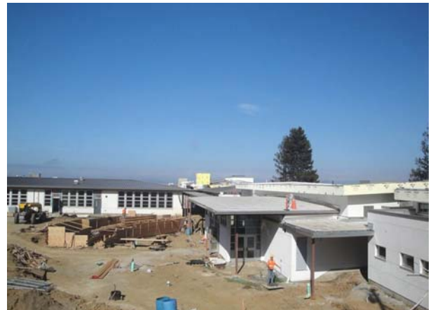
Building D - Amphitheatre form work and rebar installation
