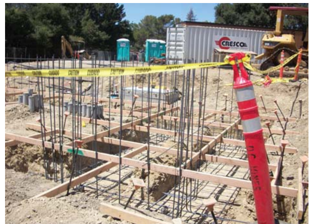
Enclosure rebar footings
