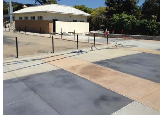
Home Locker Room and adjacent site concrete
