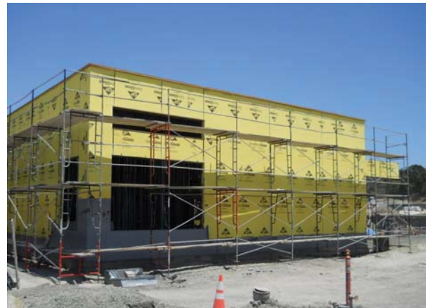
Scaffolding at Building 10 perimeter
